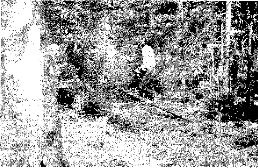
Figure 9. Cutting balsam fir to prevent shading of tube and pipe lines.
